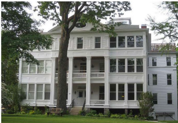
A small apartment building designed to look like a large house.
