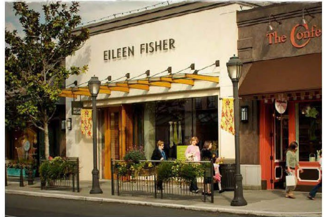
A single-story commercial building with a generous ceiling height.
