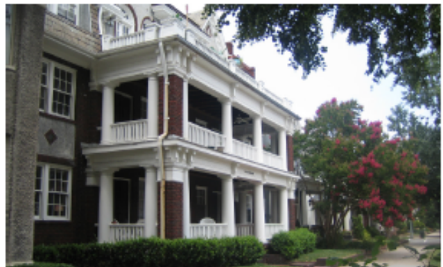
A 2-story porch on an apartment building.
