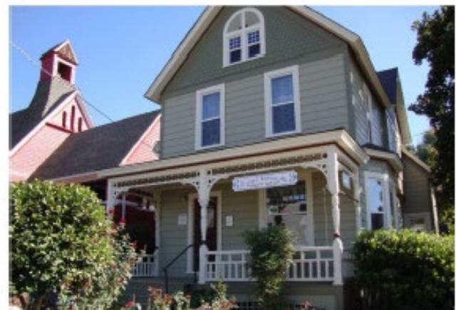
A single-family house structure containing a business.
