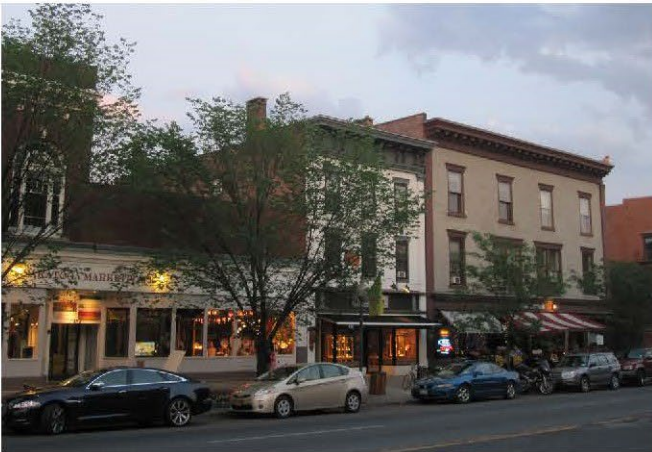
A street of commercial block buildings of varying heights and widths.
